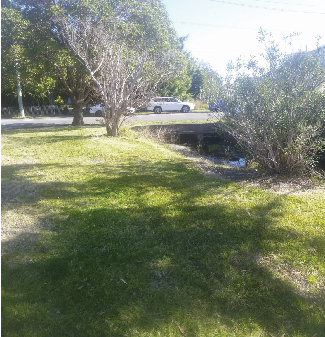
Photograph 3 – downslope of Edgar Street crossing looking upstream
