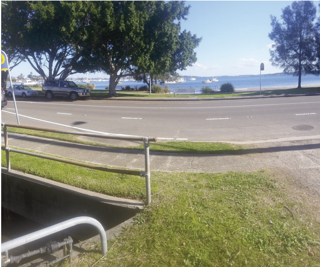
Photograph 6 – upstream of Brooks Street crossing looking downstream
