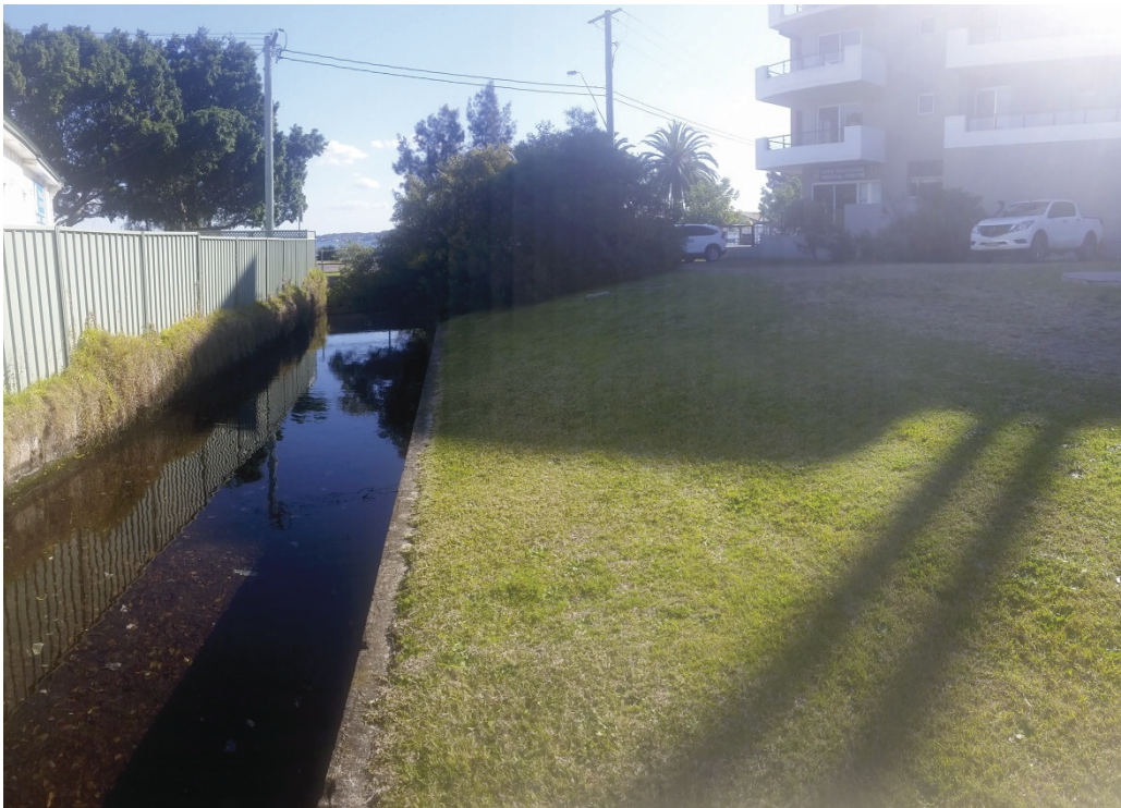
Photograph 5 - to the north of the site looking downstream
